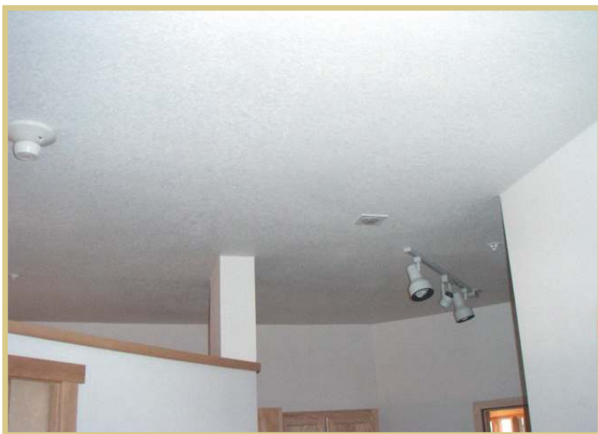
Figure 1. A typical view of a resident's ceiling, which includes a smoke alarm, IR sensor, sprinkler heads, and track lighting. All rooms also have monitoring switches on doors and stationary movement sensors. Although some features, such as the track lights, have wall switches, they are controlled through programmable logic controllers.
