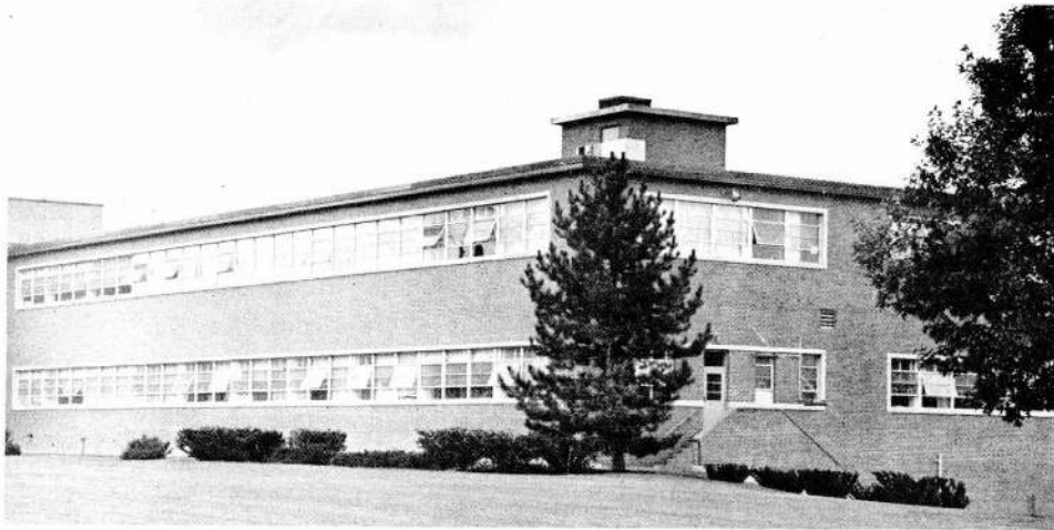
Figure 6. Northeast corner of USACRREL building. Arrows point to wall surface heated by radiators.
