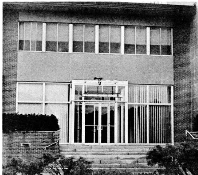
Figure 3. Main entrance of USACRREL building. Black horizontal arrows point to south-facing slate wall. White horizontal arrows point to east-facing slate wall. Each of six vertical arrows points to window with an installed storm sash.
