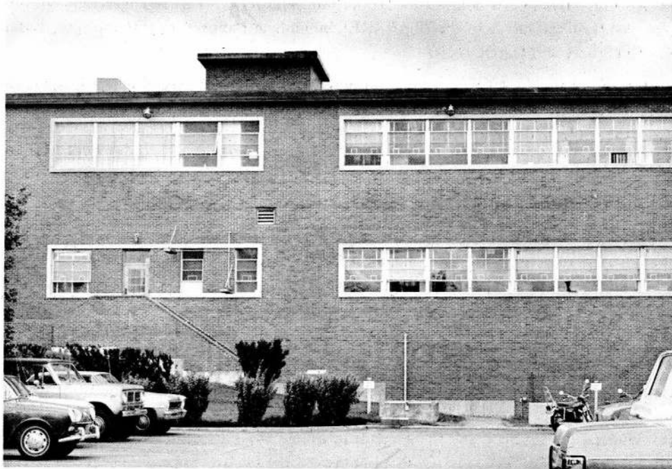
Figure 1. Northeast side of USACRREL building. Windows are numbered to distinguish differences in heat loss. (See text.)
