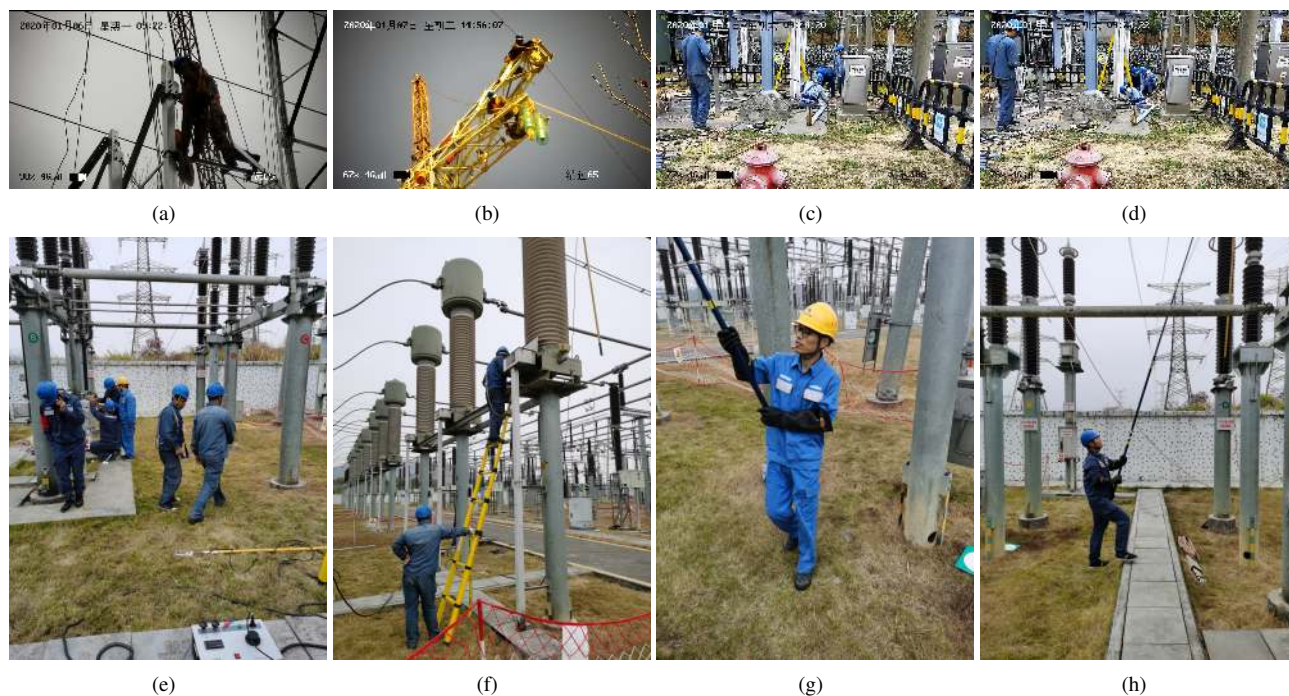
FIGURE 3. Typical samples of substation operation monitoring image dataset.
