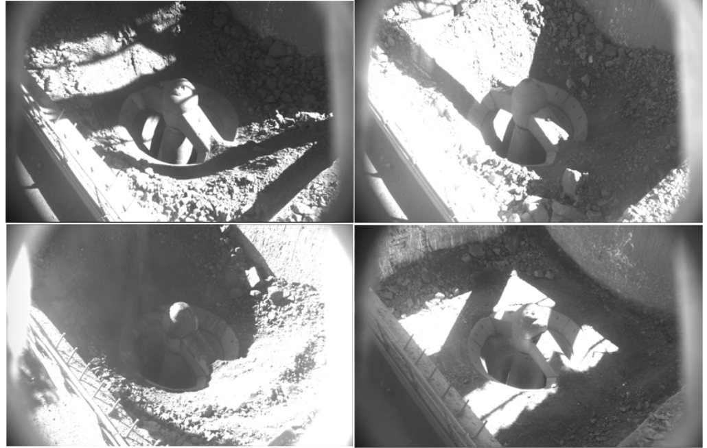
Figure 11. Crushing mouth blockage false alarm.
