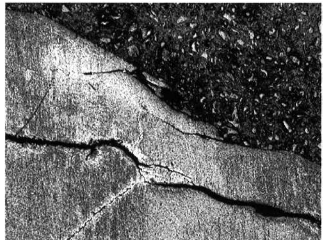
Fig. 26 Subsurface crack close to pit
