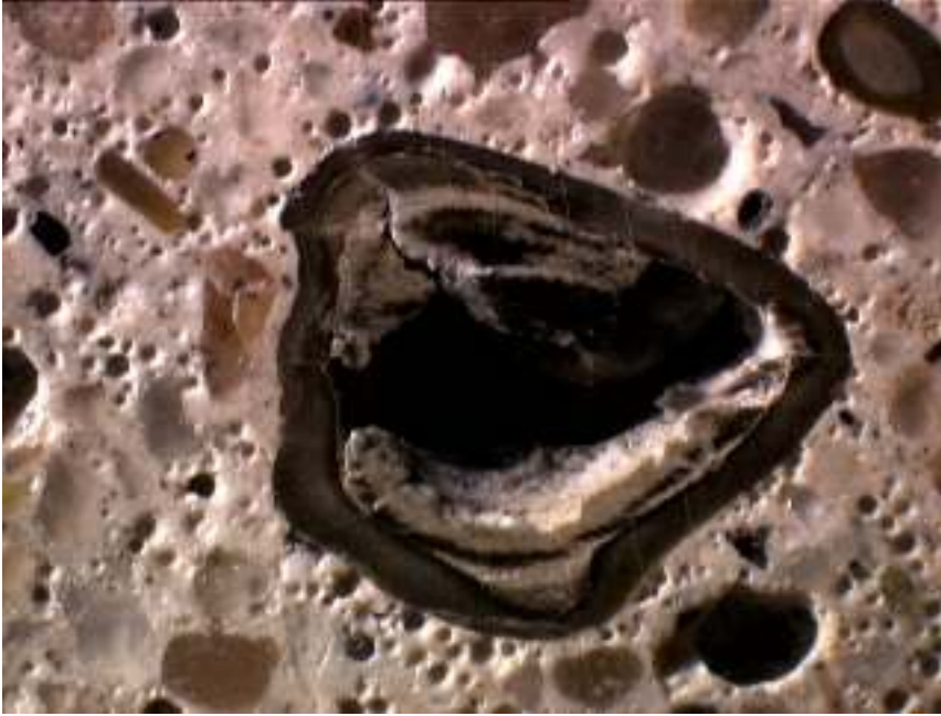
Figure 29. Core 18 mortar microstructure includes numerous shale fragments that appear to have undergone alkali-silica reaction, however little cracking of the mortar was evident. SEM examination indicated that some of the reaction product permeated the paste filling the capillary voids adjacent to the shale. Field width: 10 mm.
