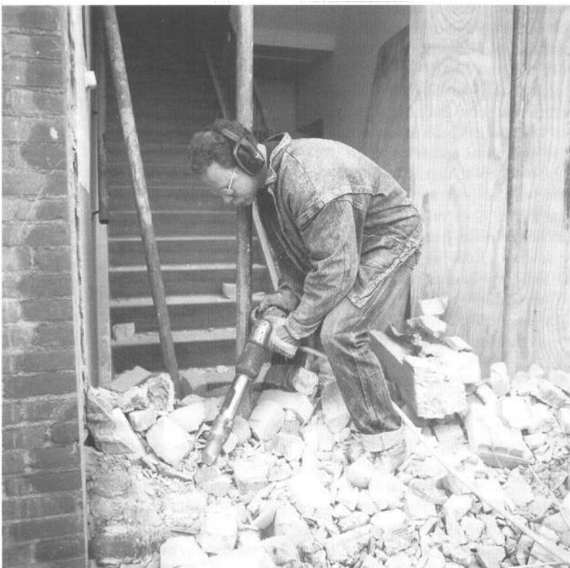
Fig. 2. A demolition worker.
