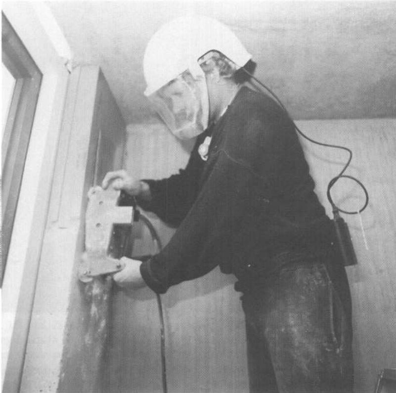
Fig. 1. A recess miller at work.
