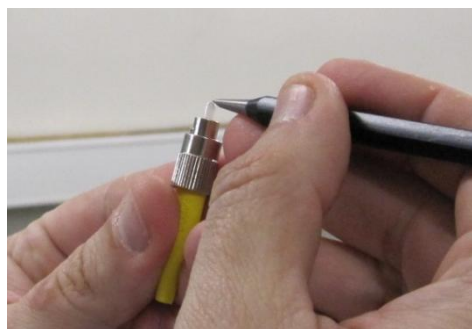
Figure 56- Scoring the optical fiber.
