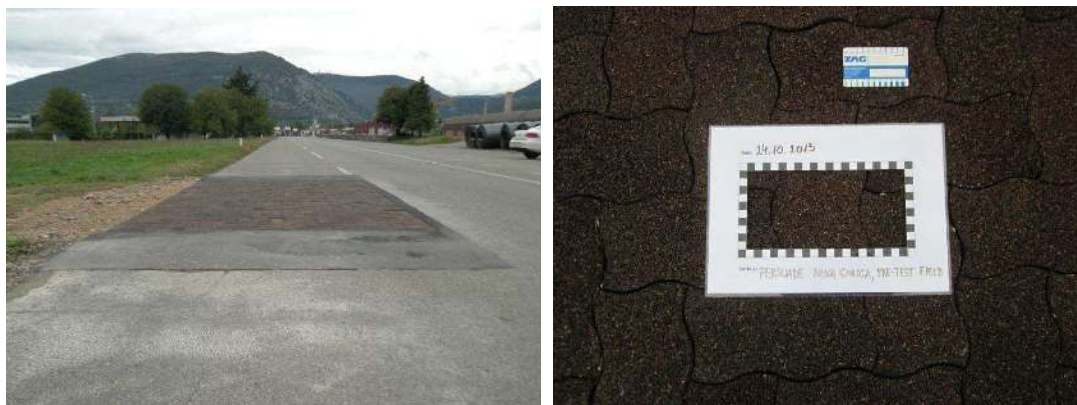
Figure 4 – The Slovenian pilot test track in Nova Gorica; prefab PERS on concrete setts (pictures: D. Kokot, ZAG)
