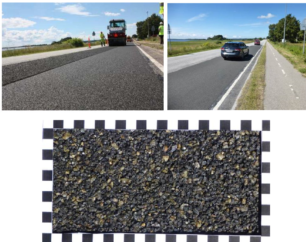
Figure 6 – The second full scale test track in Kalvehave, Denmark, built in June 2014 (pictures by H. Bendtsen, DRD). Each square in the frame is 10x10 mm.
