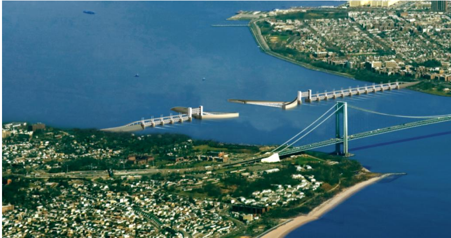
Figure 12. Conceptual Design of a Storm Surge Barrier in NYC. Source: Aerts et al., 2009
