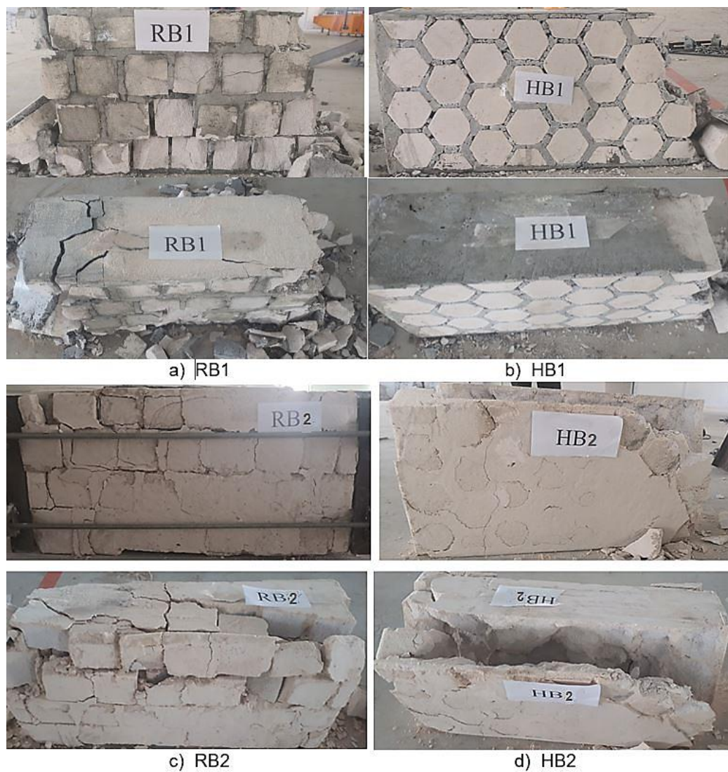
Fig. 13: Comparative views of failure modes.
