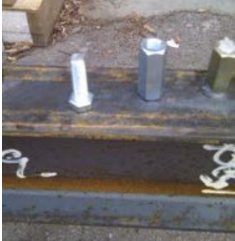
(a) Metric bolt and nut
