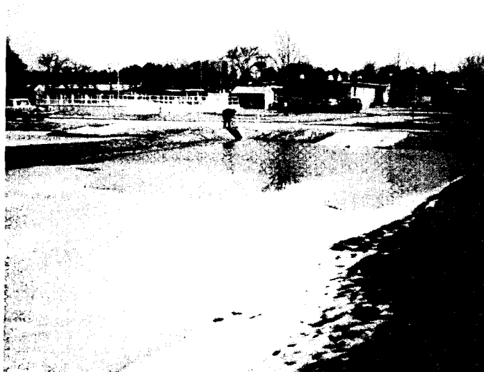
b. Sludge spreading over previously frozen layer.
