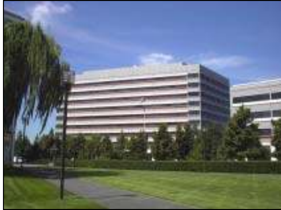
Figure 2-3. Bank of America - Concord Data Center, Building B
