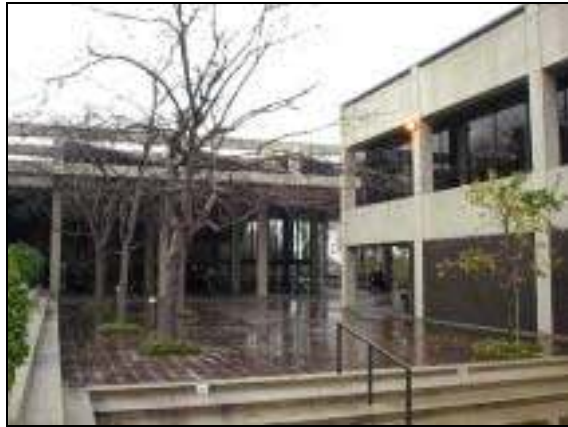
Figure 2-5. Roche Palo Alto – Building FS (left) and A2 (right)
