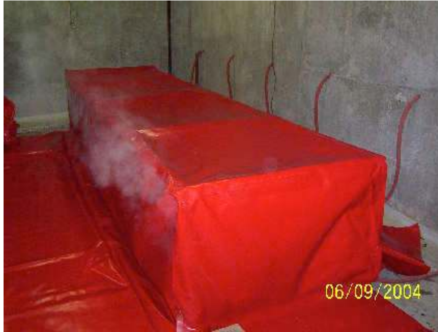
Figure 3.15: Steam Curing in Progress
