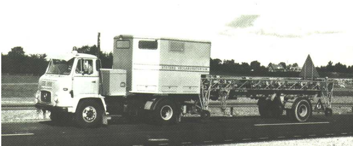
Figure 2.5: The Danish first generation Deflectograph. (Reproduced from [63].)
