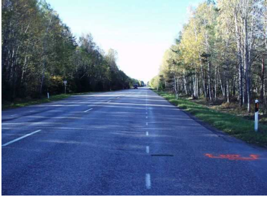
(a) Test site at Fornåsa.
