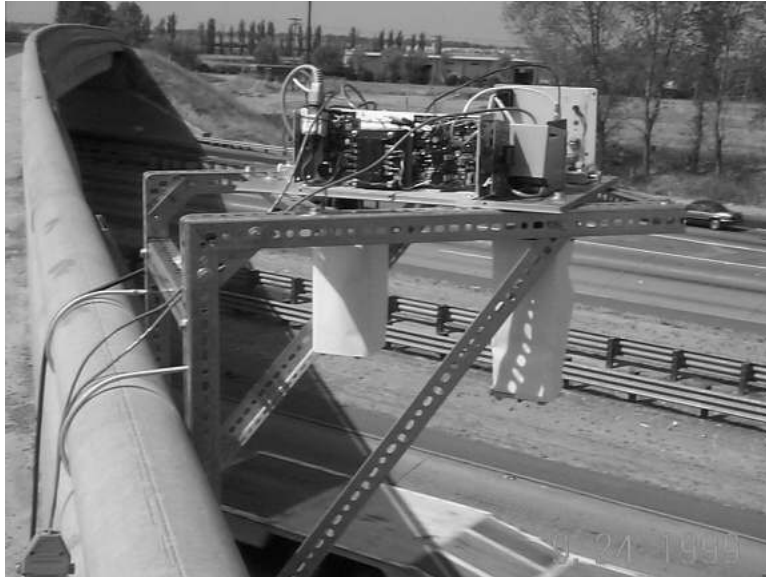
Figure 4.3: Detection system mounted above the highway
