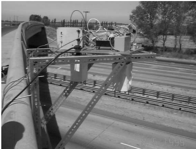
Figure 2.11: Testing prototype mounted on the cantilevered frame
