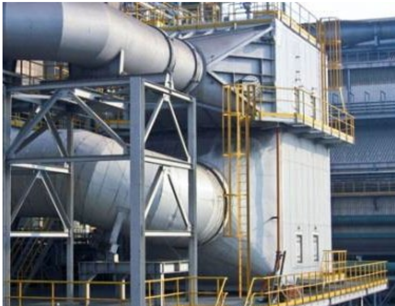
Figure 3: A functioning heat pipe heat exchanger unit.
