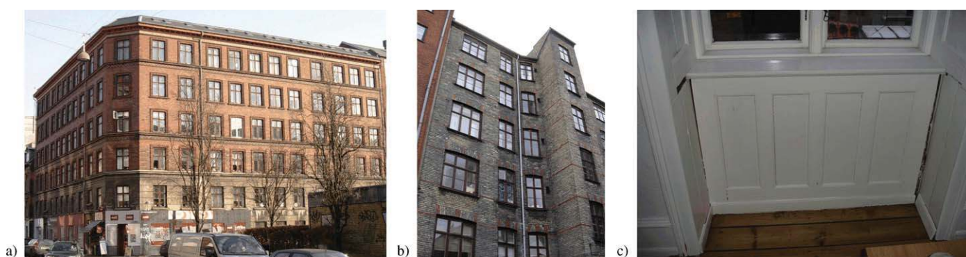
Fig. 2. (a) Street facade, (b) courtyard facade and (c) spandrel seen from the apartment.
