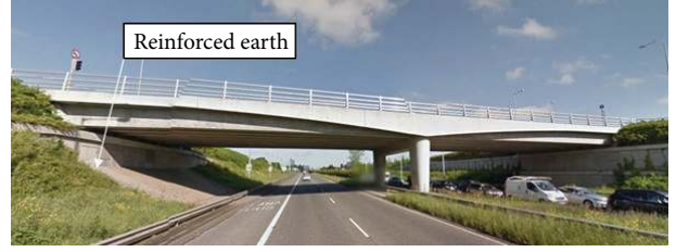
FIGURE 3: Two-span integral bridge with flexible abutment supports.
