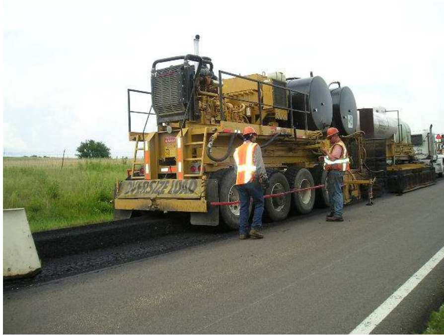
Fig. 32. Rejuvenating and mixing equipment
