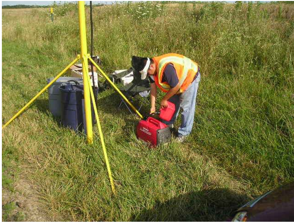
Fig. 17. Adding gas to the portable generator
