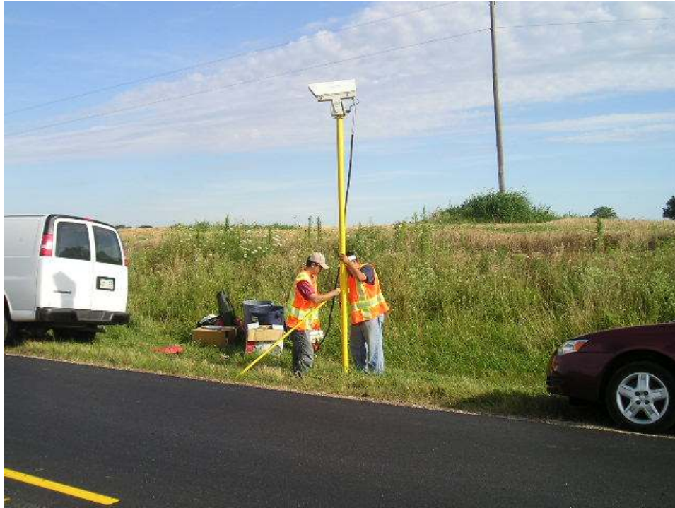
Fig. 15. Supporting the pole with three steel legs
