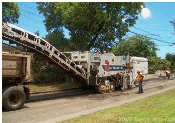
Fig. 23. Milling (Washington Asphalt Pavement Association 2002)
