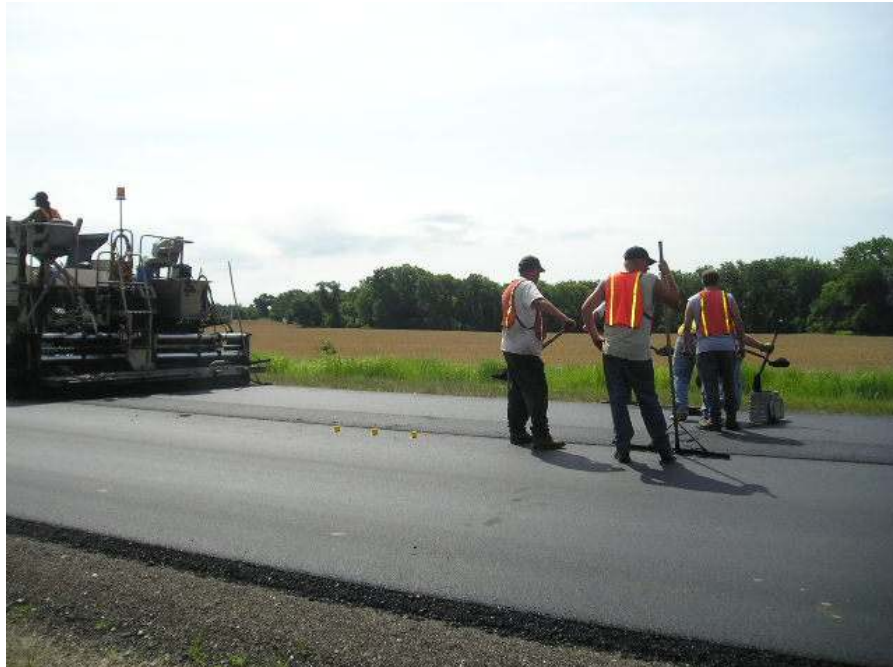
Fig. 26. Sampling the asphalt mix for lab test
