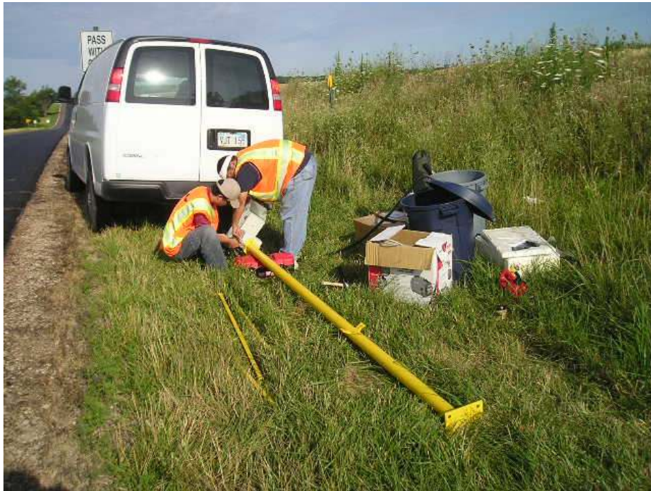
Fig. 13. Mounting camera on the pole
