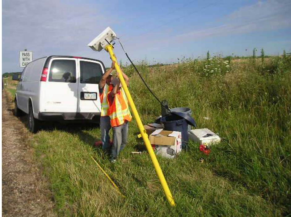
Fig. 14. Erecting the pole perpendicular to the ground
