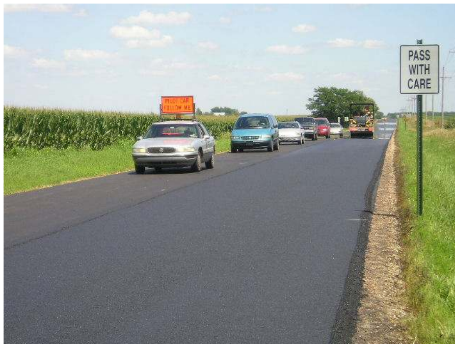
Fig. 22. Traffic control (single lane closure)
