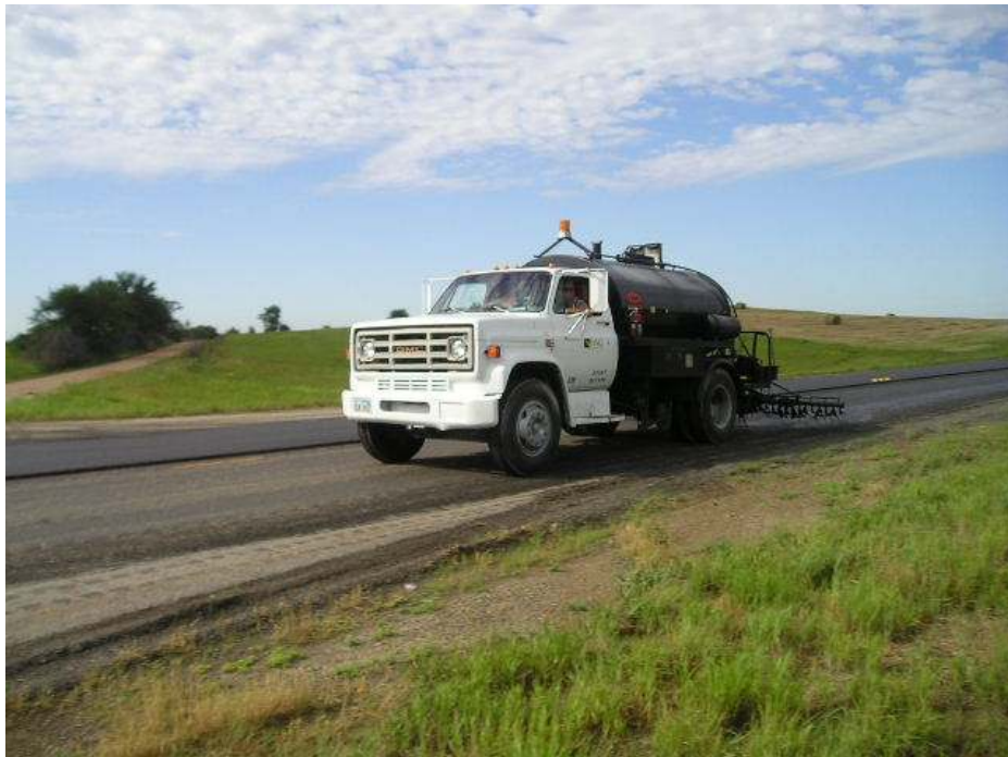
Fig. 24. Tack coat material applied by a pressure distributor
