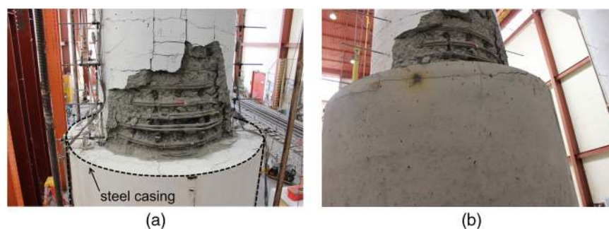
Fig. 9. Damage in Specimen 3: (a) column base and top of the pile; (b) pile after removal of the steel casing
