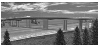
Figure 10 Dongying Yellow River Bridge in Shandong (2003, over 1800 FBGs used)
