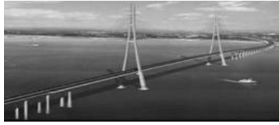
Figure 12 Nanjing third Yangtze river Bridge (2003, over 300 FBGs used)
