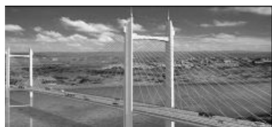
Figure 9 Songhua River Bridge in Heilongjiang (2003, over 50 FBGs uses)
