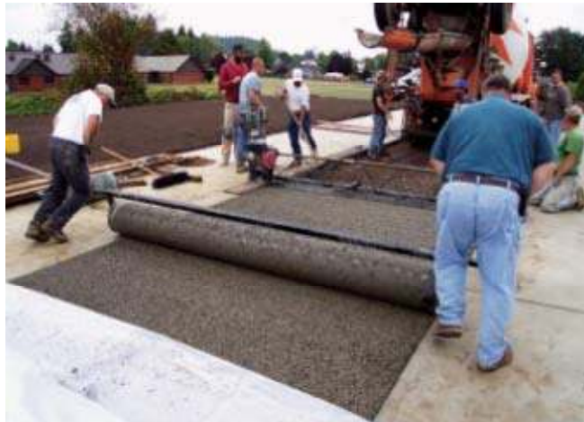
Figure 2.14: Use of a Steel Roller
