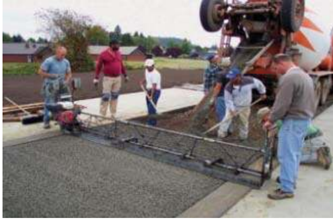
Figure 2.13: Mechanical Vibrating Screed
