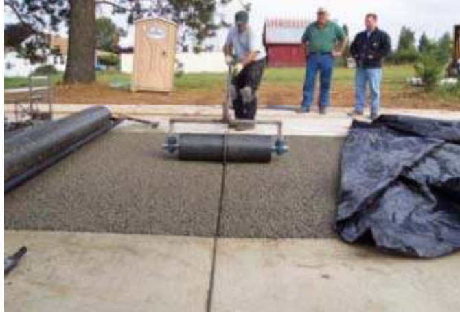
Figure 2.15: Use of a Rolling Joint Tool
