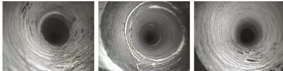
(b) After grouting (0.5 m, 1.5 m, and 2.5 m)
