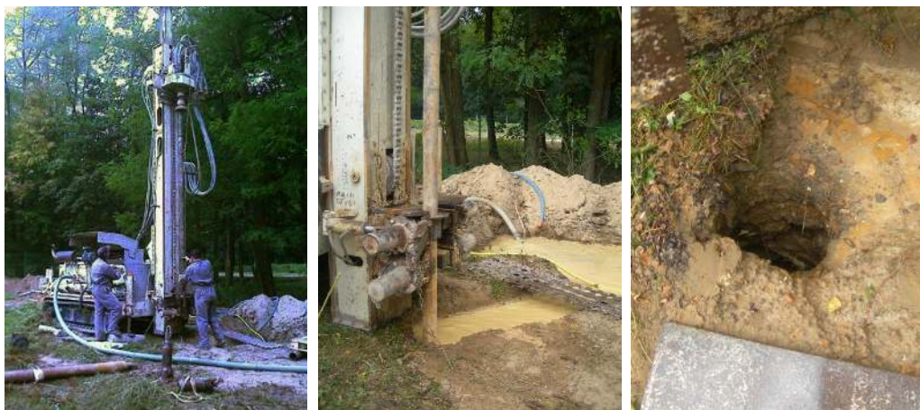
Figure 4.4: Drilling operation and borehole
