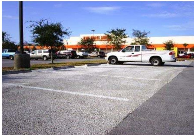
Figure 2.27 Pervious concrete parking lot [35]
