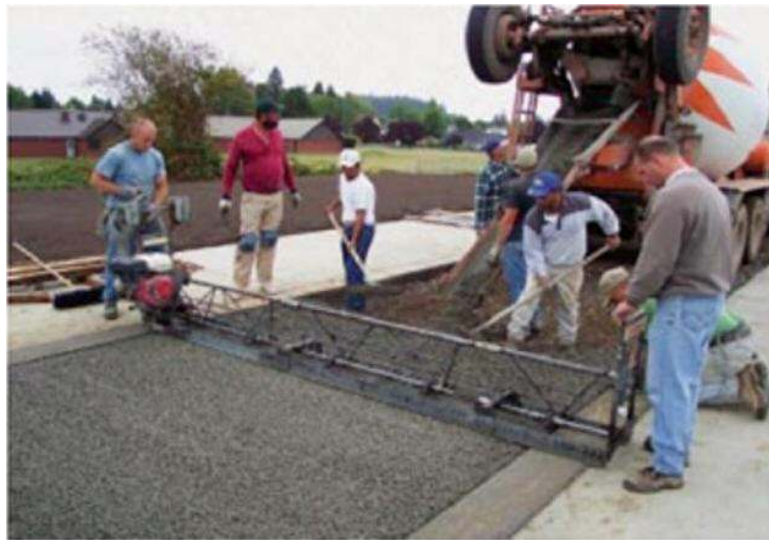
Figure 2.25 Placing pervious concrete [2]
