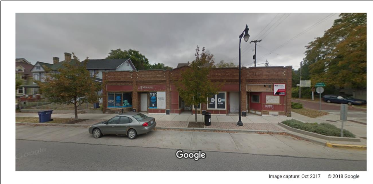
Figure 6.3: Abandoned Building at Wealthy and James St. Source: Google, 2018.
