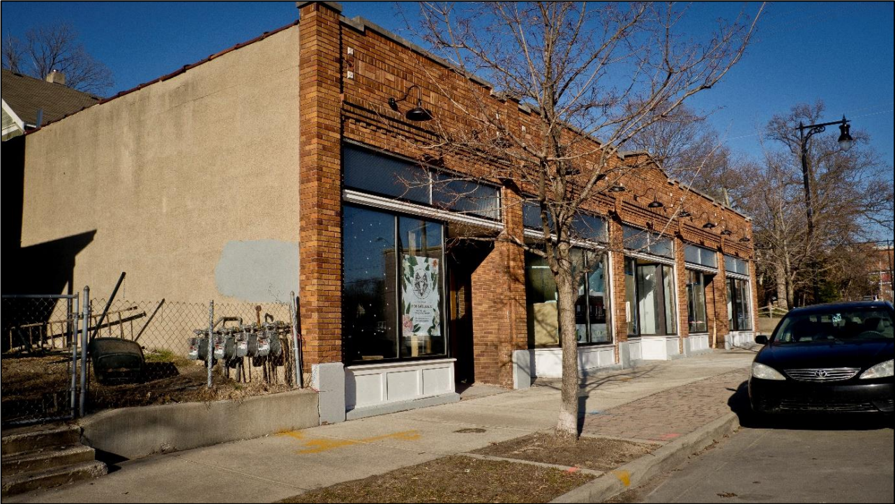
Figure 6.5: Refurbished Building at Wealthy and James St -clear of tags. Source: Author, 2018.
