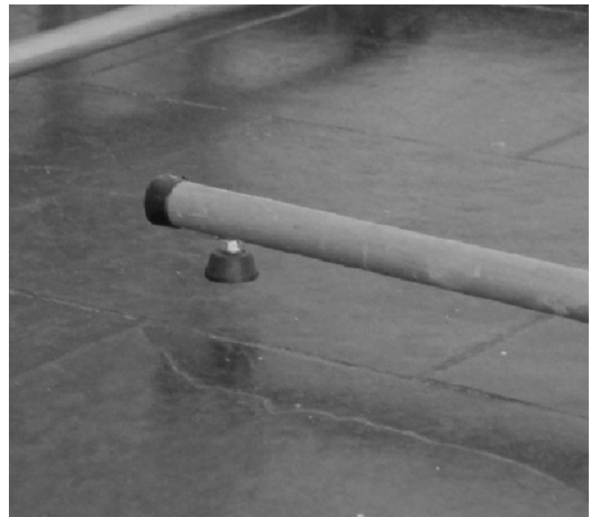
Figure 3. The small rubberized supports. Source: elaborated by the authors.
