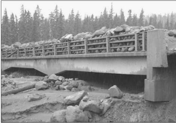
FIG. 1. The aftermath of flooding and a debris flow on the White River in OR on 7 Nov 2006. This view is of the down-river side of the White River Bridge on Highway 35, southeast of Mt. Hood. (Photo courtesy of Doug Jones, Mt. Hood National Forest.)
