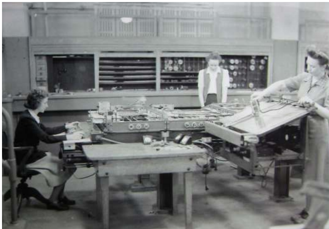
Differential Analyser for Solving Differential Equations invented 1876 built 1927
