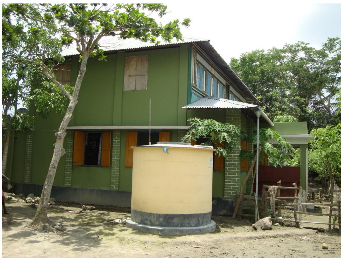
Figure 2. Rainwater-harvesting tank (4400 L) of a household in a village community in Bagerhat District, Bangladesh.
