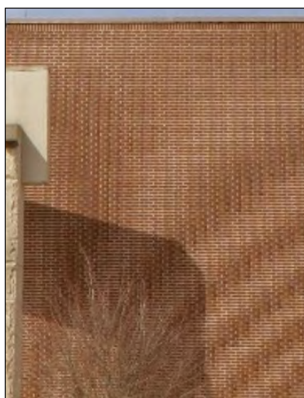
Figure 3: Aliasing of a brick wall by undersampling. Credits: This picture was provided by Cburnett on Wikipedia ( http://upload.wikimedia.org/wikipedia/commons/f/fb/Moire_pattern_of_bricks_small.jpg ).
