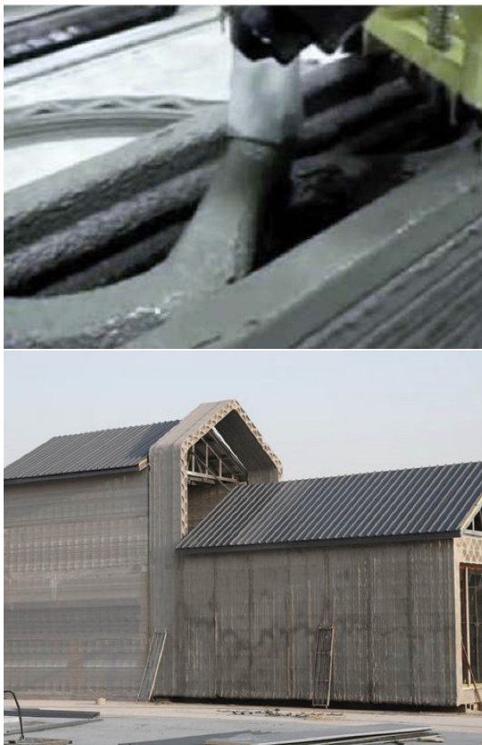
Figure 3. (Top) Contour Crafting, with layers of approximately 5 cm. (Bottom) House printed and assembled by WinSun.
