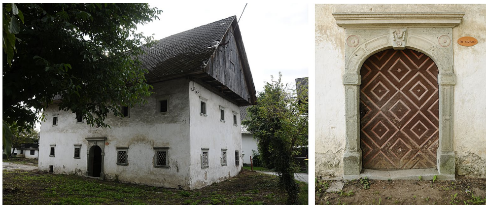
Fig. 1 Mrak's Homestead (left) and the entrance portal (right)
