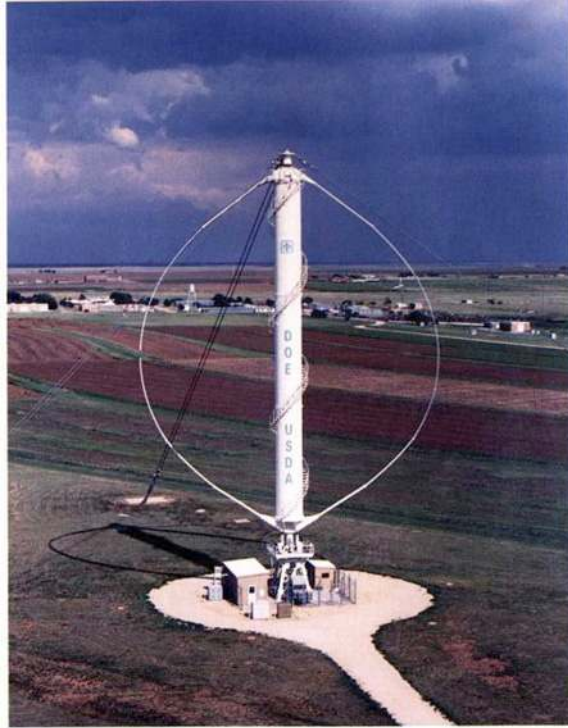
Figure 2.2: A Sandia turbine with 34 m diameter [25].
