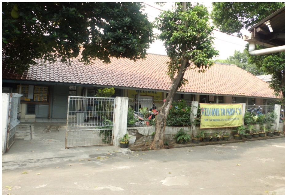
Figure 5.2 Wijaya Learning Centre building
