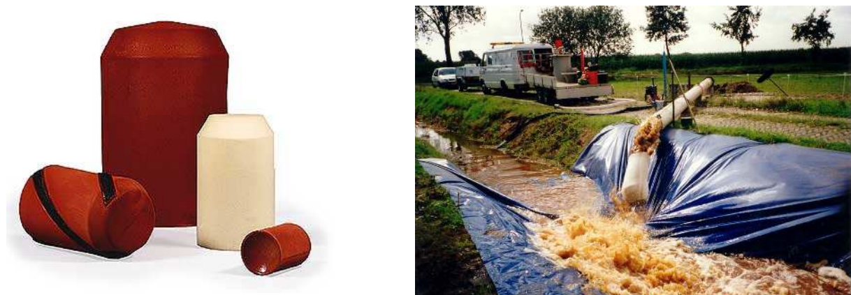
Fig 5-7 Left, some examples of pigs used in pipe cleaning; right, the outlet of pigs with a dedicated flushing point
