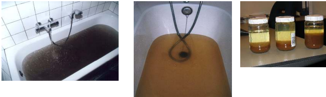
Fig 1-2 Examples of discoloured water
