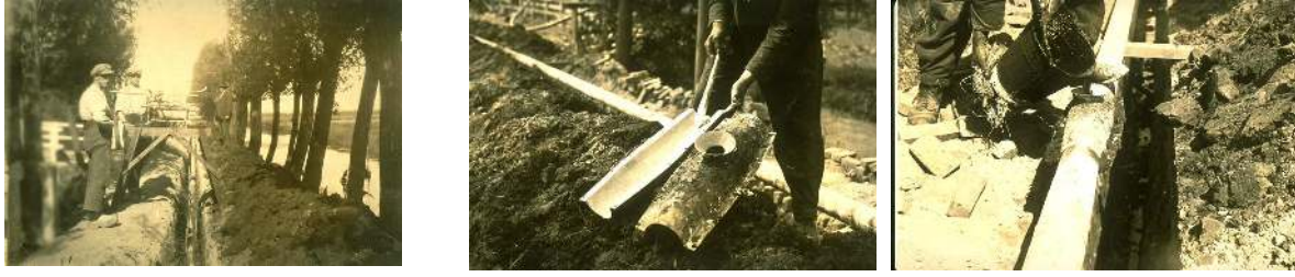
Fig 7-1 Pre-1940 pipe laying with lead joint
