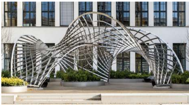
Fig. 1 The INSIDE-OUT pavilion by Schling and Hitrec on the campus of TU Munich. (image: Felix Noe)
