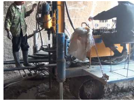
FIGURE 5: Construction of vertical jet grouting piles.
