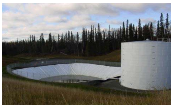
Figure 8. The landfill leachate collection pit [46].
