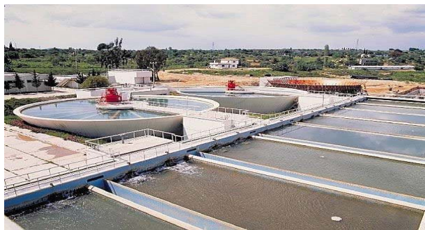
Figure 15. Filters used to treat pesticide wastewater through adsorption [89].
