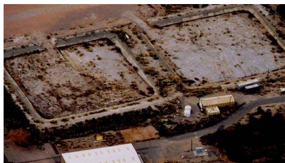
Figure 6. Evaporation beds for disposal of pesticide wastewater [43].
