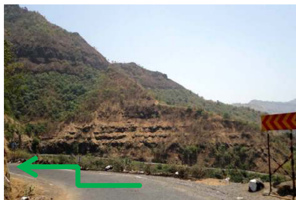
Figure 1. The panoramic view of the hill slope.
