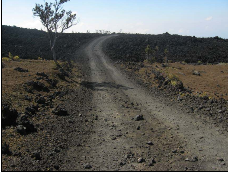
Figure 1.10. Location of the western margin of the Argentine ant population along the road above Hawaiian Ocean View Estates Subdivision on the Kahuku section of Hawai`i Volcanoes National Park. Cinder (light substrate in foreground) supported ants while the adjacent historic-age `a`ā flow (dark substrate in background) did not support ants.
