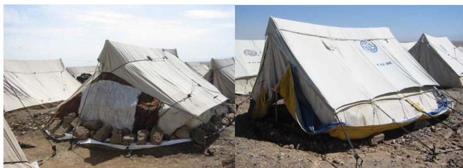
Figure 4 Canvas ridge tents illustrating (4a) draft blocking and (4b) ventilation by occupants (Maslack, March 2002)
