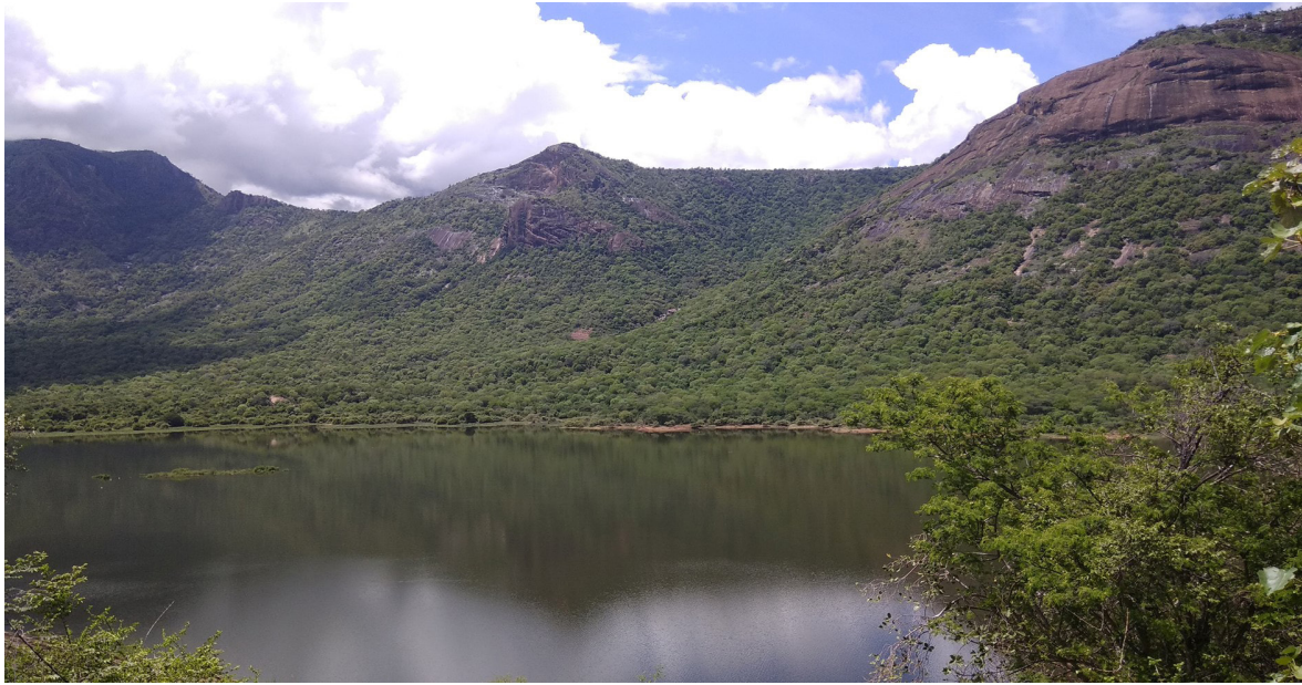
Figure 2. View of Pilavakkal Dam
