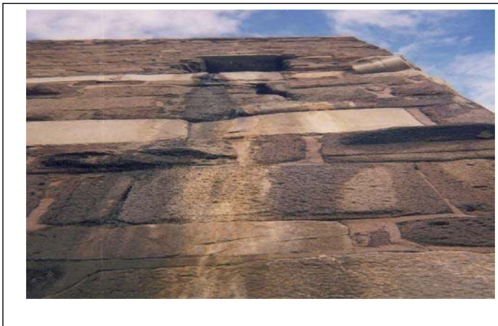
Figure 3.2 A view from north elevation at Gençkapı Gate; salt depositon and alveolar weathering on the andesite surface
