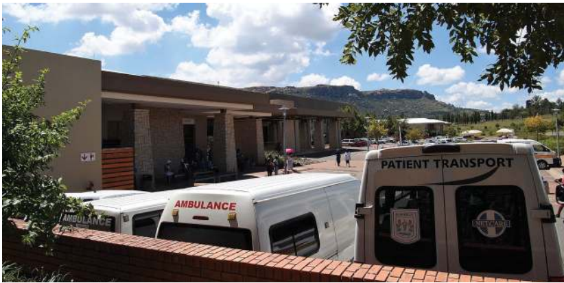
Photo: The Queen 'Mamohato Memorial Hospital in Lesotho. Experience with this hospital highlighted problems of investing in hospital care without a strong primary health care system. Photo from the collection of Patrick Smith, used with permission. More at: A dangerous diversion: Will the IFC's flagship health PPP bankrupt Lesotho's Ministry of Health? OXFAM Briefing Note, 7 April 2014.
