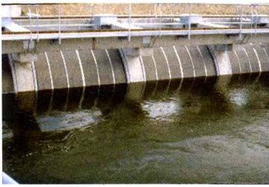
Photo 1: Conventional drum screens at an irrigation water intake in USA.
