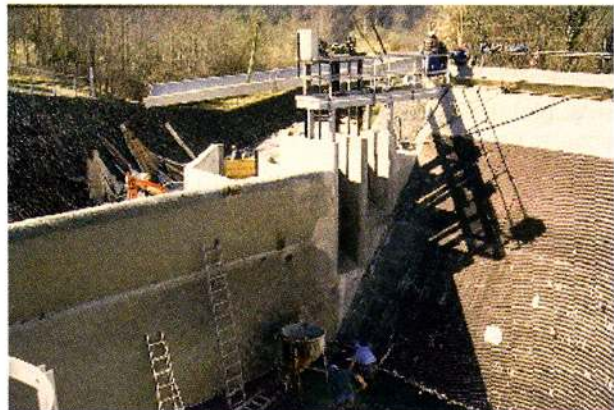
Photo 11: Surface bypasses at the power intake of St Cricq scheme (Gave d'Aspe river, Pyrenees). Note the two entrances at different elevations.
