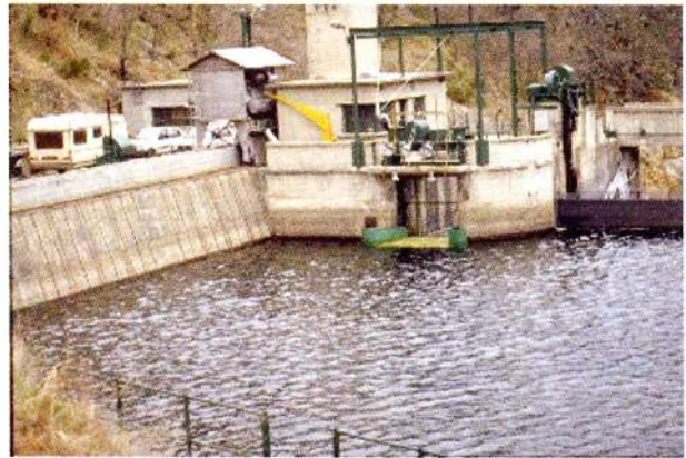
Photo 9: Downstream surface bypass at the Poutes dam (Allier river). The 10 m deep power intake is located on the left.
