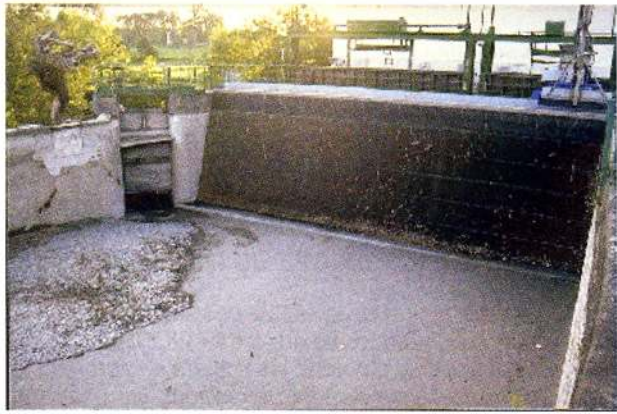
Photo 8: Downstream surface bypass at the Soieux power station intake (Gave d'Aspe river, Pyrenees).
