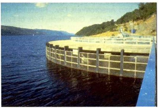
Photo 2: Fine mesh screens at a pump storage hydroelectric intake in Scotland.
