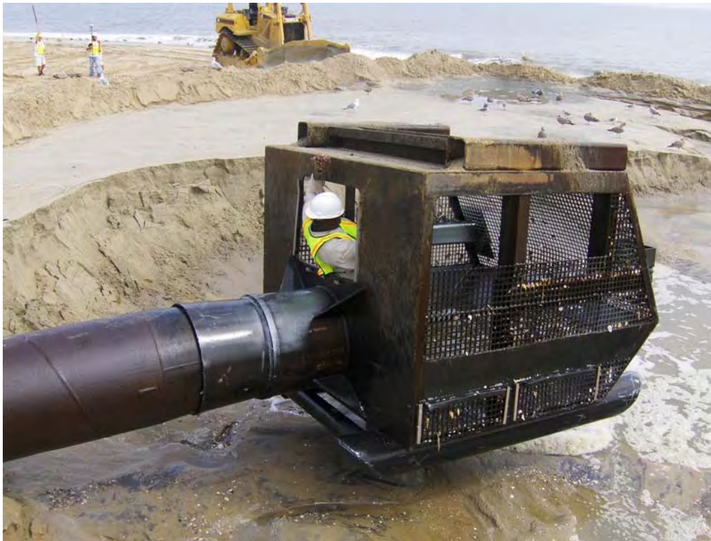
Figure 39. UXO Specialist inspection of beach screening basket at Bethany Beach, DE (2007).
