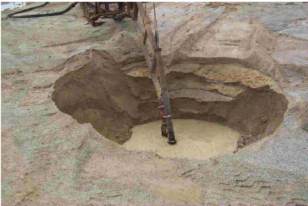
Figure 17. Eductor-formed excavation crater.
