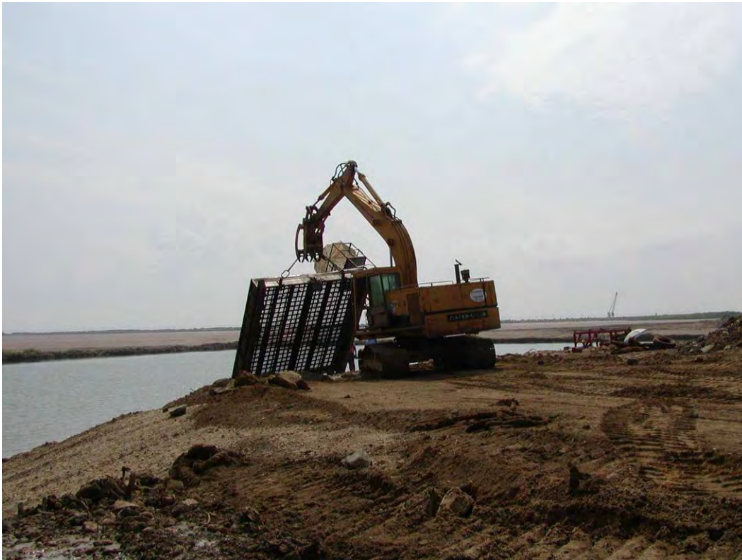
Figure 88. Clearing debris from HMI static screen.
