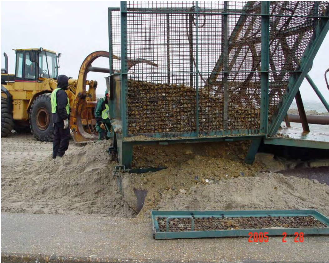
Figure 75. Trap door removed from discharge basket screen.
