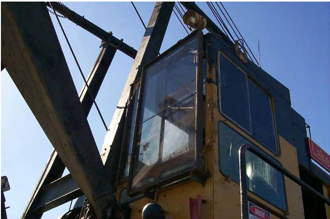
Figure 111. Crane operator's protective barrier.
