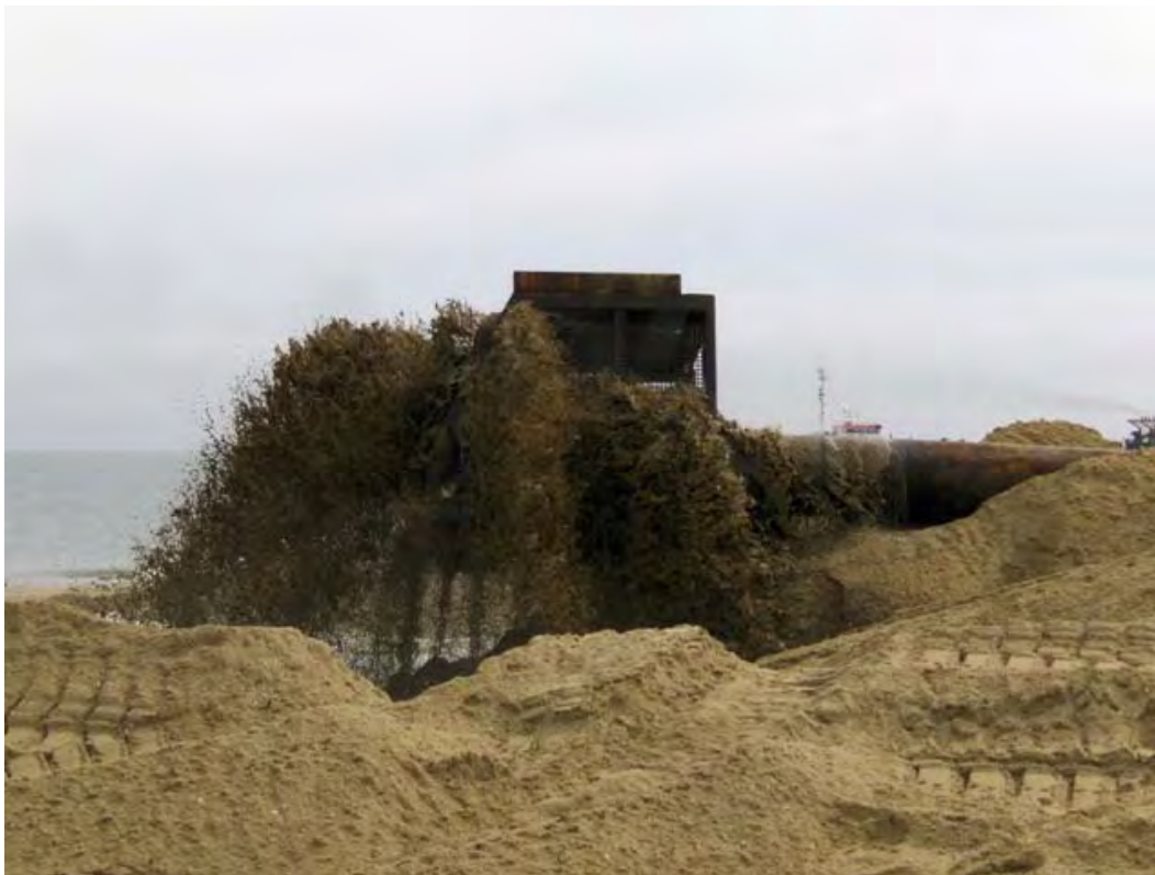
Figure 38. Beach screening basket in operation at Bethany Beach, DE (2007).
