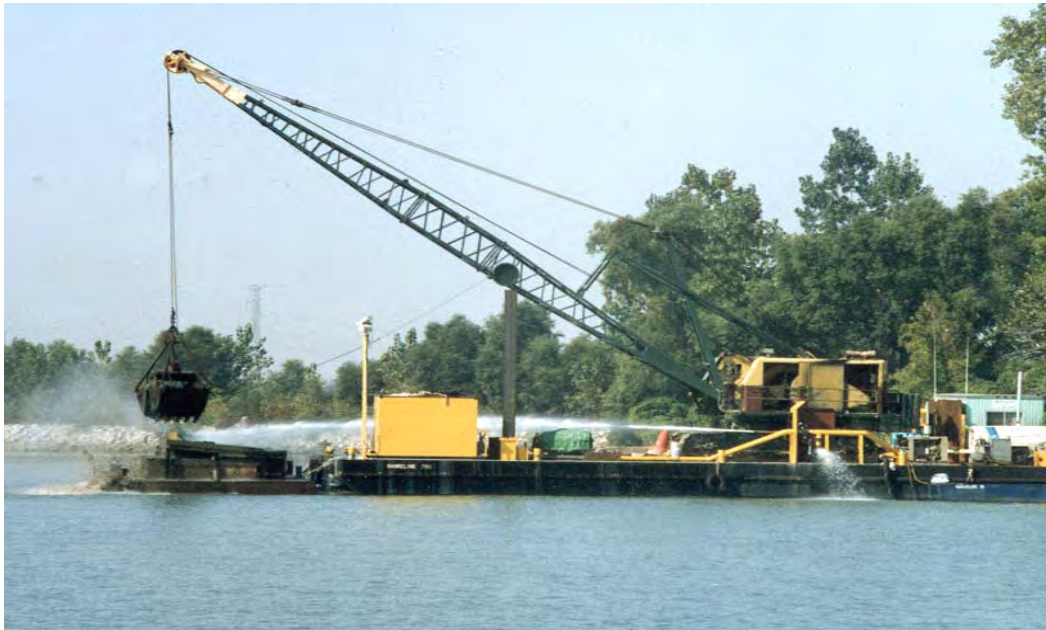
Figure 98. Deck layout and MEC dredging system (courtesy of Shoreline Contractors, Inc.).
