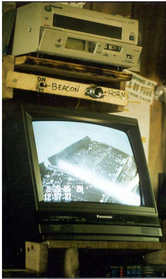
Figure 103. Closed-circuit television control station inside observation trailer (lens zoomed out).
