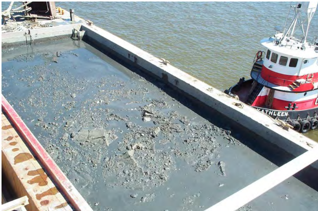
Figure 77. Barge ready to be hydraulically unloaded at HMI.
