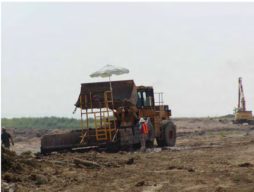
Figure 85. Front-end loader placing debris on HMI static separation screen.
