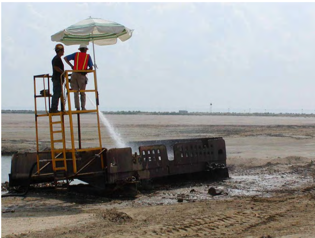
Figure 87. Application of water jet on HMI static screen.
