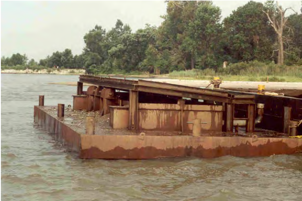
Figure 99. Scow and separation screen.
