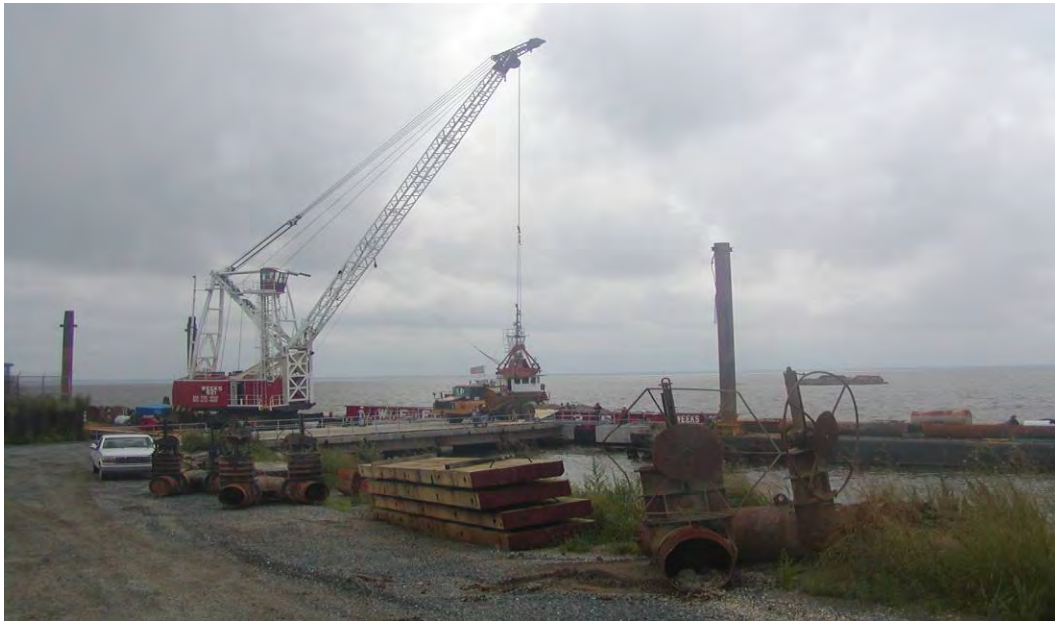
Figure 82. Unloading debris from barge bottom with clamshell bucket.
