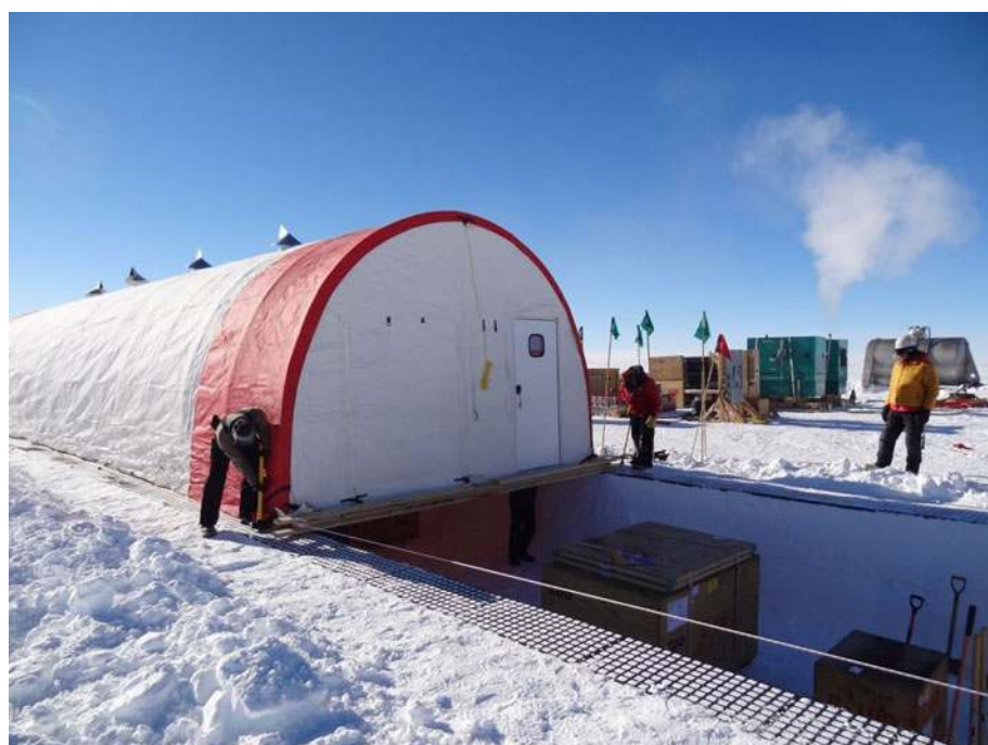
Fig. 2. IDD tent being pulled into place over the drill trench.
